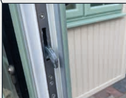
Multipoint door locking system with high security euro locks on all our doors
